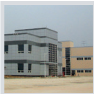
Wuxi Plant (China)
