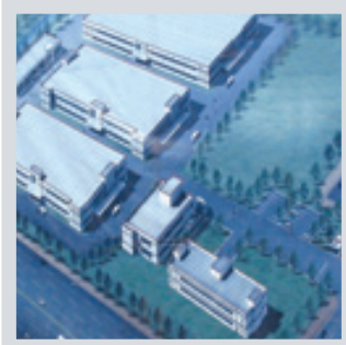
Wuxi Plant (China)
