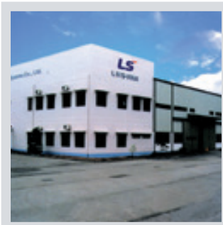
Hanoi Plant (Vietnam)
